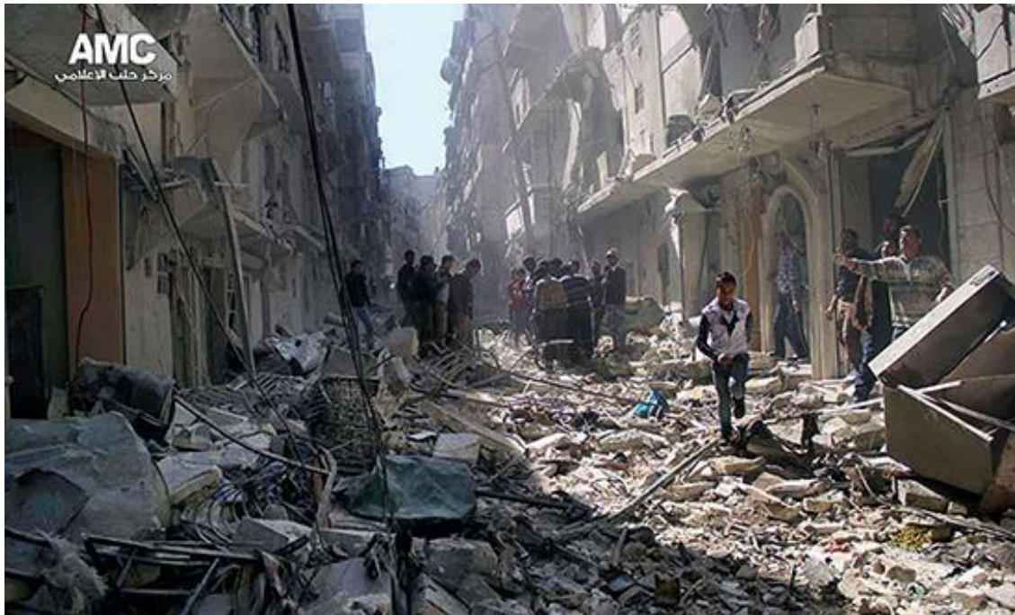
Figure 1. Syrians inspect the rubble of destroyed buildings following a Syrian government airstrike in Aleppo, Syria on 19 March 2014 © AP Photo/Aleppo Media Center AMC.
